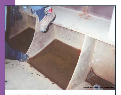
Residual water accumulated at lowest point of an upper wing tank.
